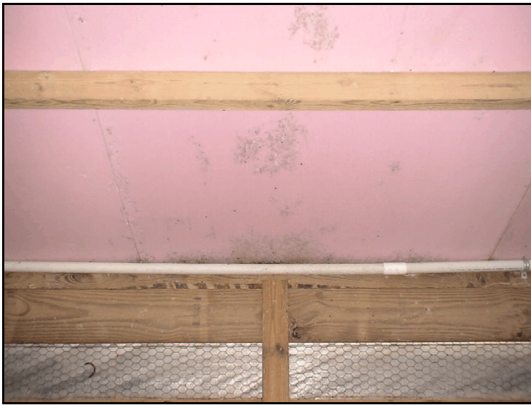
Figure 13. Beetle damage of polystyrene insulation. Dark spots are holes where beetles have burrowed into the insulation.
