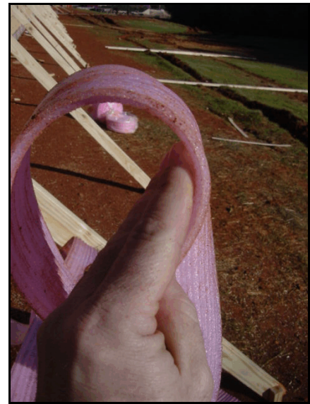
Figure 14. New sill sealer.
